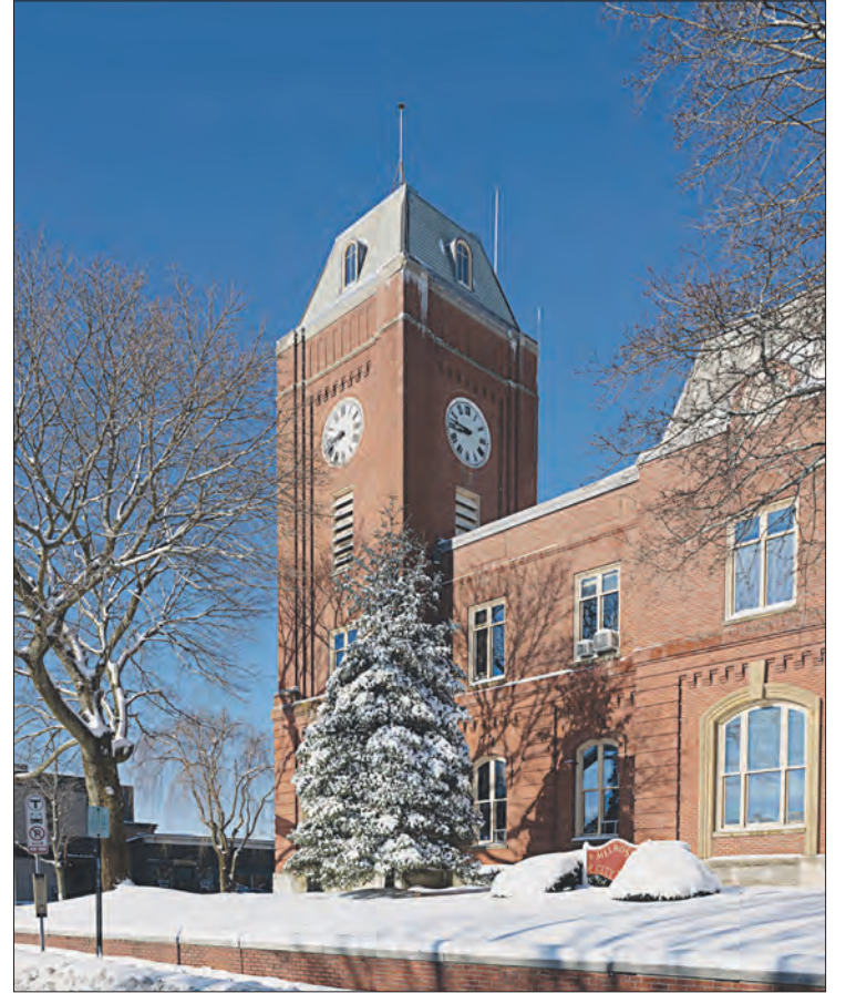
AFTER LAST WEEK'S winter storm went out to sea, City Hall stood out against a cloudless blue sky.
